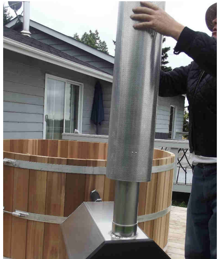
Fig. 10.2.3 Assembling the heater stack.
