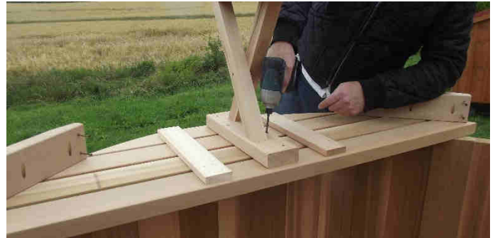
Fig. 10.1.2 Attach bench brackets with supplied 2" screws.
