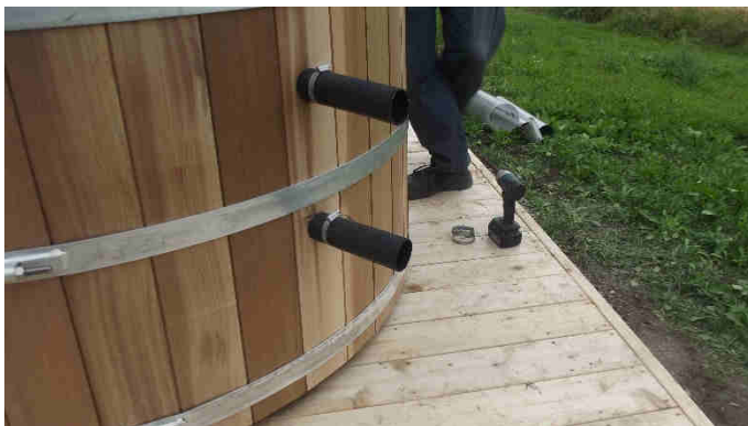
Fig. 10.2.2 Attach heater hoses with gear clamps
