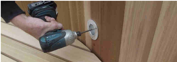
Fig. 10.2.1 Fasten heater hose fitting.
