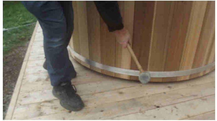
Figure 9.1 Hitting staves directly on the strap.
