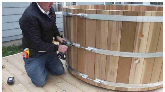
Figure 9.3 Using power driver to tighten. Stop when you see noticeable deflection of the aluminum blocks. This indicates bottom strap is tight enough. Upper straps should not be as tight.
