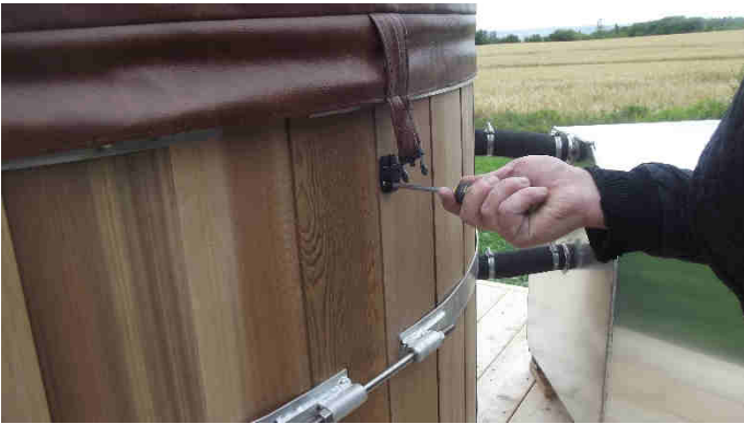
Fig. 10.4.1 Attaching the cover strap buckle.
