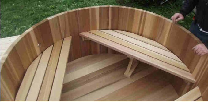
Fig. 10.1.4 Position the benches so that no screws will be driven into any seams between staves.
